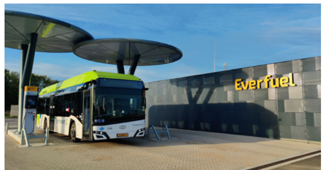
Hydrogen refuelling station near the Connexion bus depot in Heineoord (Zuid-Holland).
